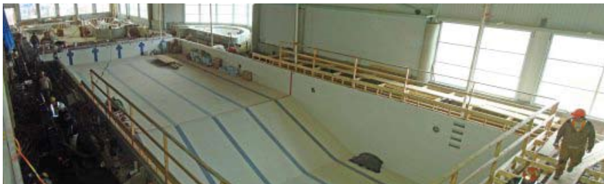
Creating the lazy river and southwest wall of the leisure pool.
