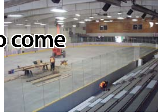
Finishing touches on CDCC arena project.
