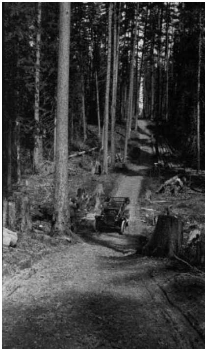
Lister-Porthill Road about 1916.
