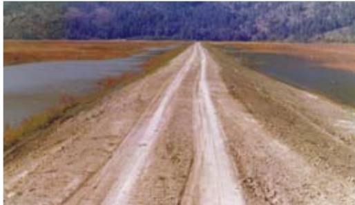
A newly constructed dike in Leach Lake in 1975.
