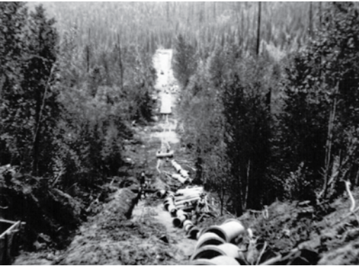
Cement pipe being laid during construction of the Arrow Creek Irrigation System, 1930.
