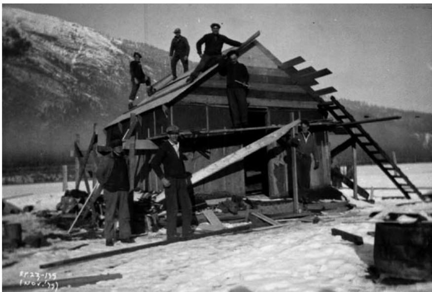
Sleeping hut near Kitchener airport.
