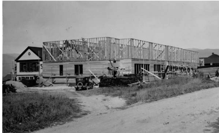
Creston Valley Junior-Senior High School under construction, 1938. Photo taken by Guy Constable, a member of the building committee
