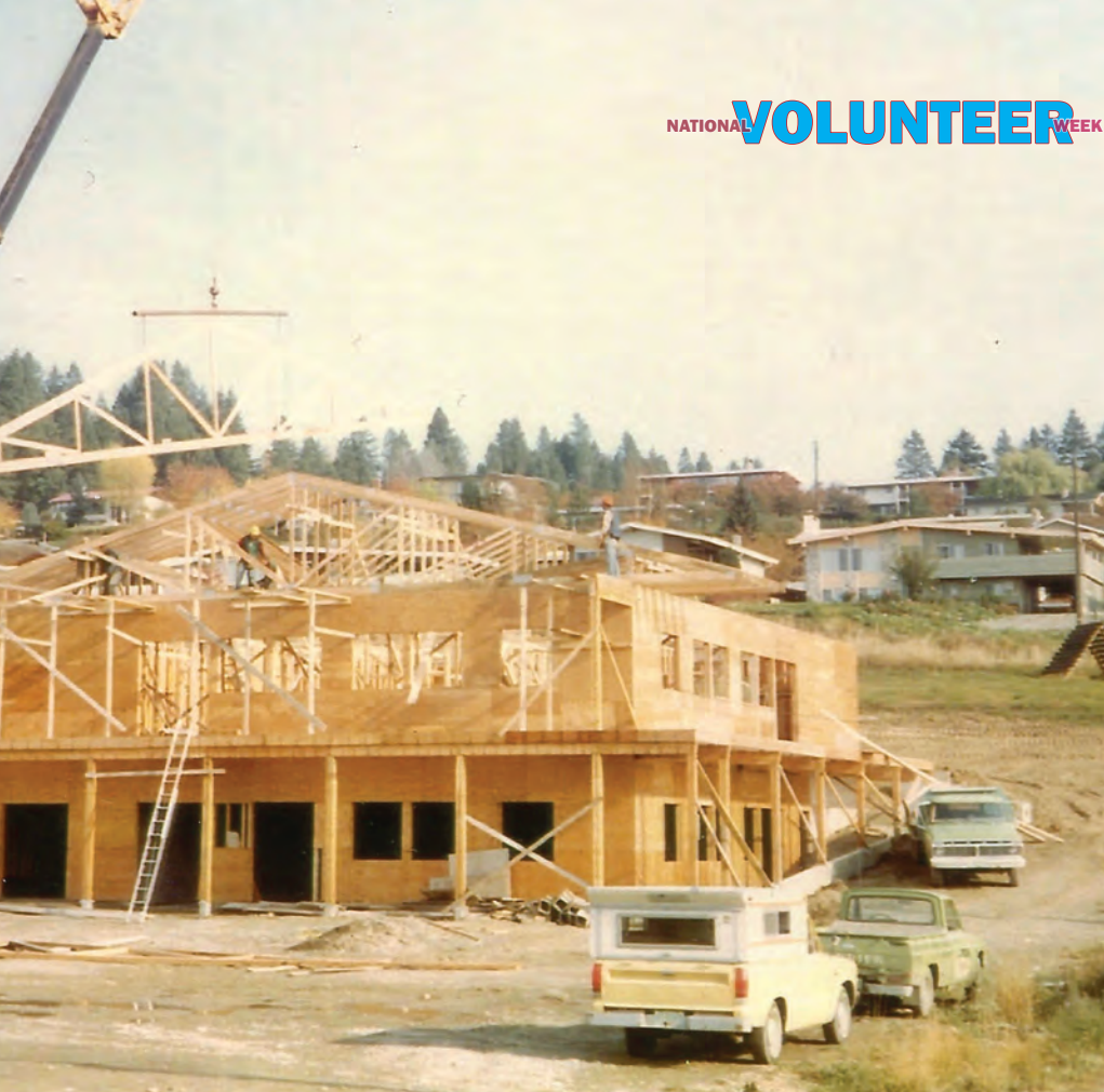
Photo submitted by: Mike Stutter Early construction of Rotacrest Hall.
