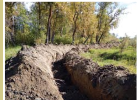
A dike being excavated for rodent runs.
