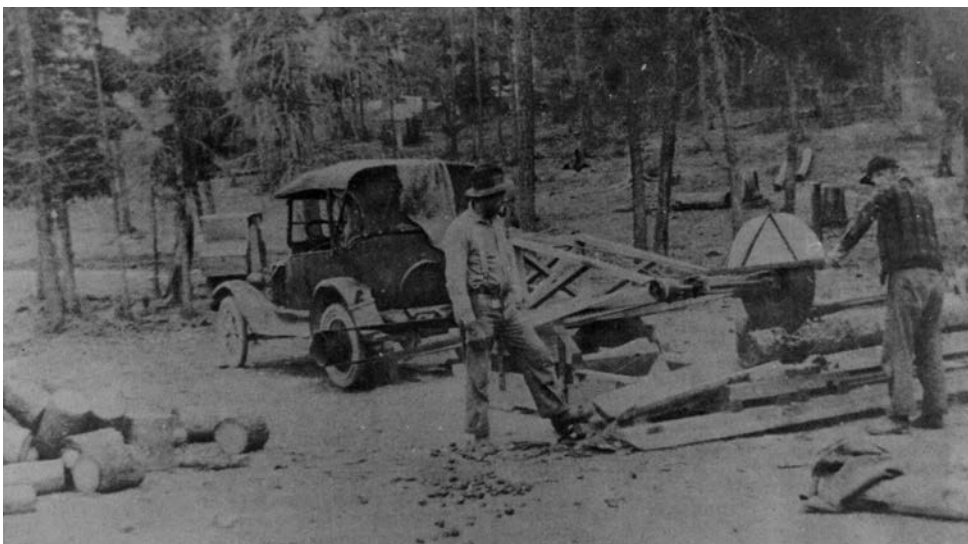
PHOTO: On the ingenuity of forest workers: Harry and Bill Demchuk cutting firewood, Lister, 1935, using a manual saw powered with a belt running off the rear wheel of a 1921 Overland car.
